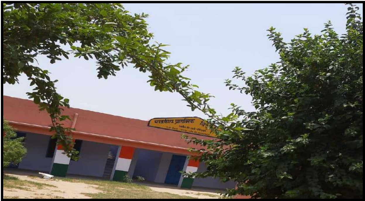
White-wash of school building of Govt. Primary School, Aasin ki Dhani, Dhiryawas.
